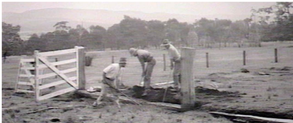
Oban Soldier Settlement – erecting gates. (Government Printing Office –Trove)
